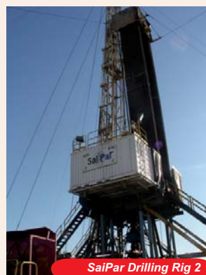
SaiPar Drilling Rig 2
